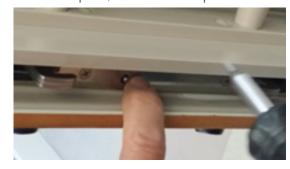
6. Compress the strike pin and activate the locking hardware.
