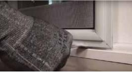
3. To reinstall the screen, line up the top two wheels back inside the track and push up the screen as high as it will go. Hold the screen out slightly and push the wheel up with the putty knife and slide the screen back into the track. Do the same on the other side.
