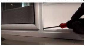
2. Next raise the screen and locate the wheels, the wheels are located at either end of the screen. Place the putty knife under the wheel, push in and lift. Once the wheel is up, gently slide the screen towards you. Do the same on the other side.
