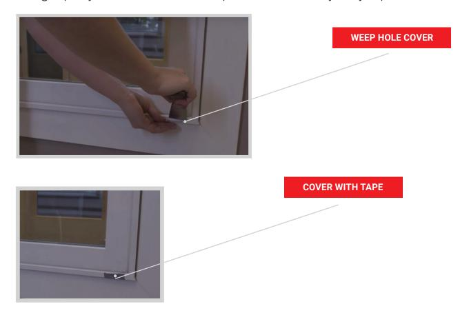
4. Fill the track with water until it is filled half way up the track edge. Let the water rest for at least 15 minutes. If there is no change in the water depth, there is no defect in the weep system.
