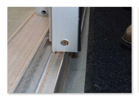
**3.** Lift up on the vent frame and swing the bottom out. Once the vent frame is removed take off any sill caps. (if any)
