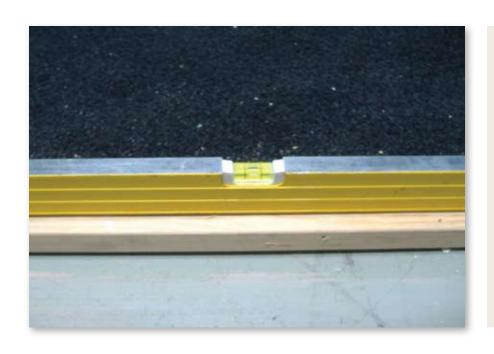
9. Check the sill for level using the longest level that will fit in the opening. Shim or flatten down any humps in the sub floor. Shims are to be made of high impact plastic capable of carrying specified compressive loads. The Horseshoe type is adequate for this application.
