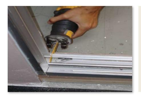
7. If you can not cut the screws, then you may cut the sill of the pre-existing door at the jambs and remove the sill so the Flush Fin door sill will set directly on the sub floor.
