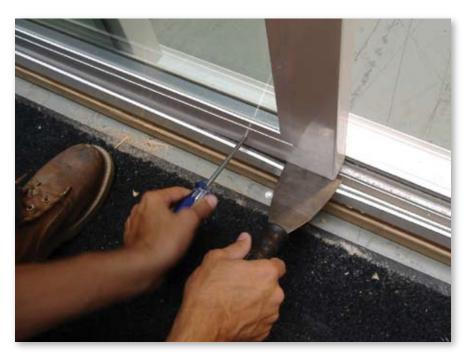
20. Remove the adjustment hole plugs on the bottom interior face of the vent frame and adjust the wheels on the vent frame. Lift up on the vent frame to take the weight off the rollers when adjusting to prevent stripping. Turn to the right to rise and the left to lower. Reveals on both sides of the vent frame should be straight. Reinstall the plugs.
