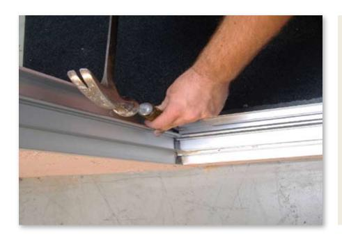
5. Using a chisel, cut through the screws that hold the sill to the jambs of the aluminum door. Use a saw to cut through the sill at center. Then remove the sill so the Flush Fin door can sit flush on the sub floor.
