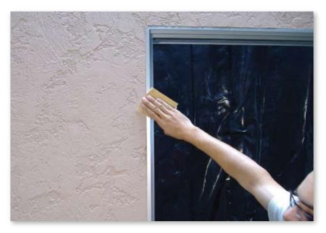
**10.** Using sand paper, scuff the pre-existing frame to ensure sealant can adhere properly.
