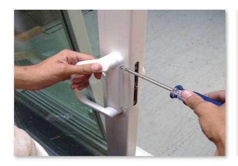
**18.** Install the supplied handle on the vent frame.
