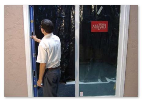
16. Check the jambs for plumb using the tallest level that will fit in the opening. Be sure to double check for square by cross measuring the door frame. Shim door frame accordingly.
