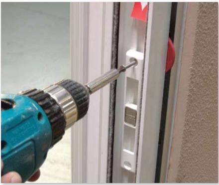
21. The strike plate comes preset from the manufacture with a screw behind the silver cover to allow for minor adjustments. Once the vent frame and strike are lined up and lockable, properly set the strike plate in place using non-corrosive screws long enough to fasten in to the framing.
