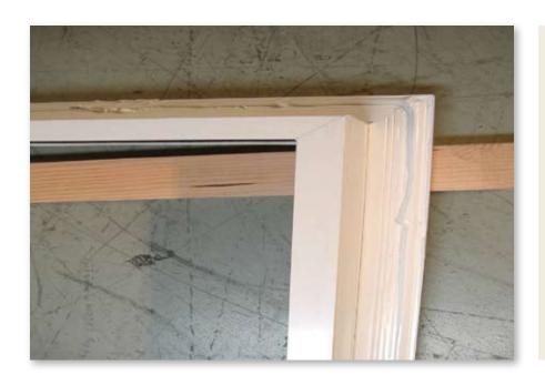
13. Apply a 3/8" diameter continuous bead of sealant (polyurethane sealant) near the back side of the outside edge of the Flush Fin. This is considered a secondary seal.
