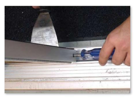
2. Remove vent frame from the Aluminum door by lowering the wheels using the adjustment screws at each end of the vent panel at the bottom (turning the screw to the right will raise the vent and to the left will lower the vent)
