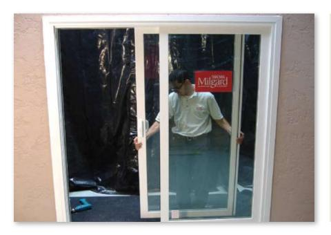
19. Install the vent frame into the perimeter frame by placing the top in first and then sliding the bottom in with the door in the open position.
