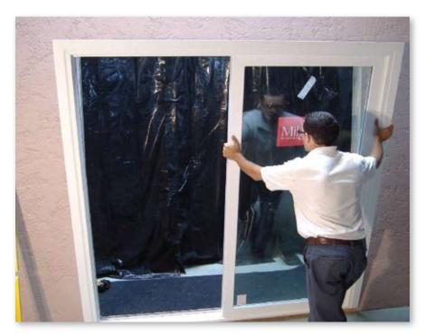
8. Check for readiness, obstructions and safety obstacles that may interfere with the installation of the door. Remove debris that will obstruct your path way during the transportation of the product. Test fit the Flush Fin retro door to ensure it is the correct size and can be installed level, plumb, and square. Remove the nail fin if not needed. Check the reveals as well.
