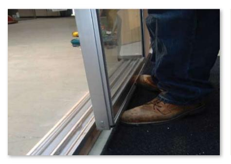
**4.** Remove any screws that are securing the fixed sash in place. Remove the fixed sash by sliding over, lifting up, and swinging the bottom out.
