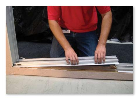
6. Once the screws are cut, you may cut the sill at the center point in order to remove the sill as shown. Do not remove the head or jambs of the original frame. Removing the frame head or jambs may damage the weather resistant barrier.
