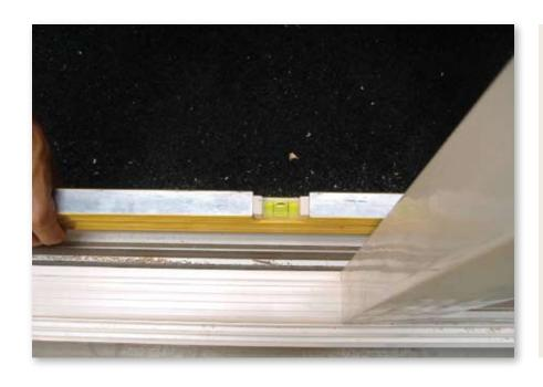
**15.** Check the sill for level using the longest level that will fit in the opening.
