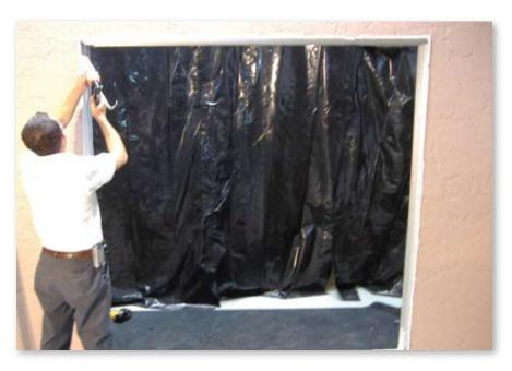
12. Apply a 3/8" diameter continuous bead of sealant (polyurethane sealant) to original perimeter frame where it will come into contact with the Flush Fin of the new door. This is considered the primary seal.
