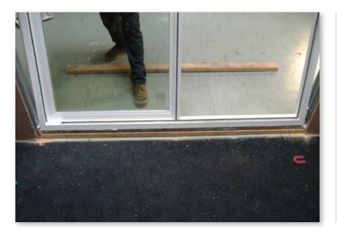
**14.** From the exterior lift the Flush Fin door and set in to the opening.
