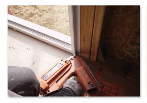
**38.** Place the side jamb extender tight against the sill of the door and fasten in place. Repeat at the other jamb.
