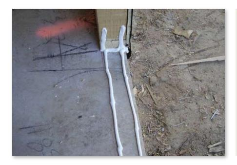
**18.** Caulk sub sill with 2 – 3/8" diameter continuous beads of sealant on the sub floor and continue 6" up the jambs.
