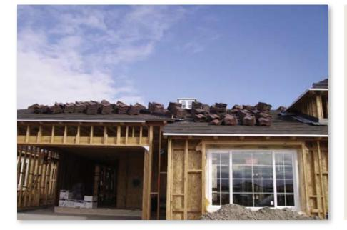
**3.** Ensure that all roofing material has been loaded on roof prior to installing.
