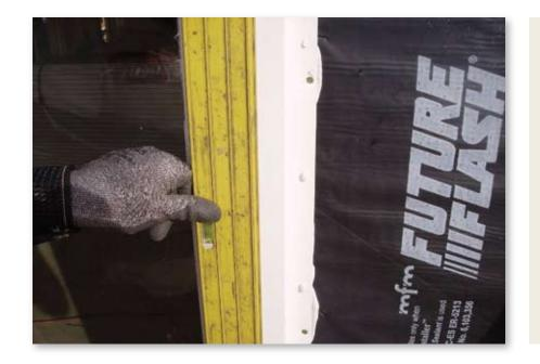
**31.** Secure the door with the fasteners at a maximum distance of 16 inches on-center. It is critical that you verify for plumb and straightness within the jambs for every two fasteners put in place.
