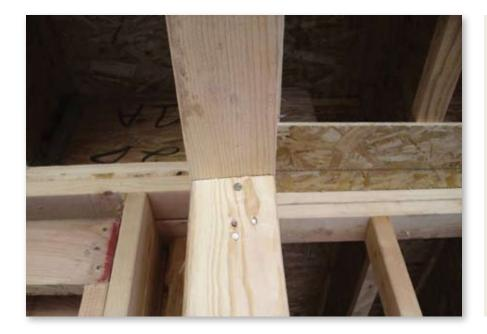
**15.** Be sure that the header and the trimmers are lined up and flush to each other.
