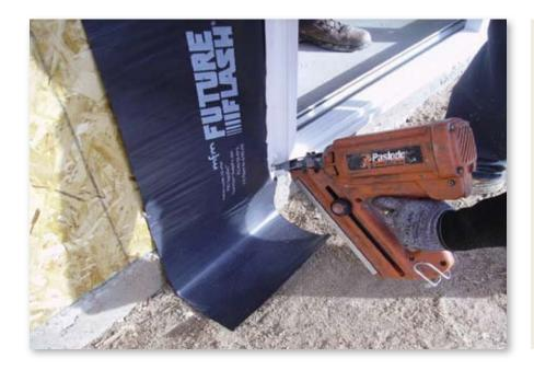
**30.** Once the door is square and plumb, fasten the door in place at the opposite diagonal corner. (Lower left corner to upper right corner and lower right corner to upper left corner.) Check the scope of work for proper fasteners.
