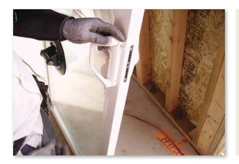
**42.** Install the supplied handle on the vent.
