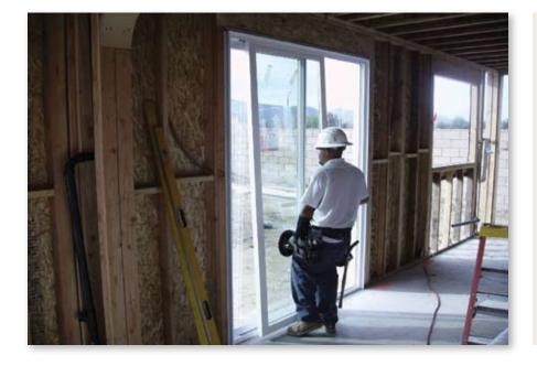
**43.** Install the vent into the perimeter frame by placing the top in first and then slide the bottom in.
