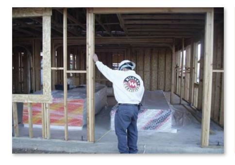
**13.** Check the **height** by measuring the vertical distance at the left, middle and right side of the opening.
