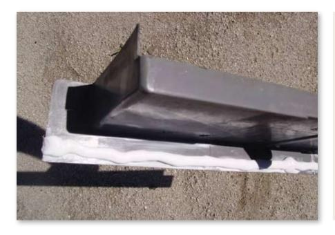
**20.** Apply one 3/8" diameter continuous bead of sealant on the bottom of the sill pan located to the back side of the down turned leg.
