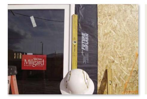
**29.** Check the jambs for plumb, both inside and outside, using a 6-ft. level or longer.
