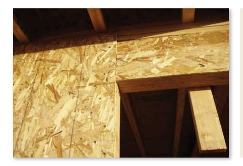
8. Check to see if the sheer panel is in place on the entire exterior opening and the same thickness is all the way around (if applicable).
