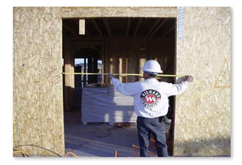
**12.** Check the **width** by measuring the horizontal distance at the top, middle and bottom of the opening.
