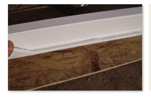
26. Apply a 3/8" continuous bead of sealant around the full perimeter of the back side (interior surface) of the mounting flange. Alternatively, you may apply this bead to the opening where the nail fin comes in contact with the flashing material.
