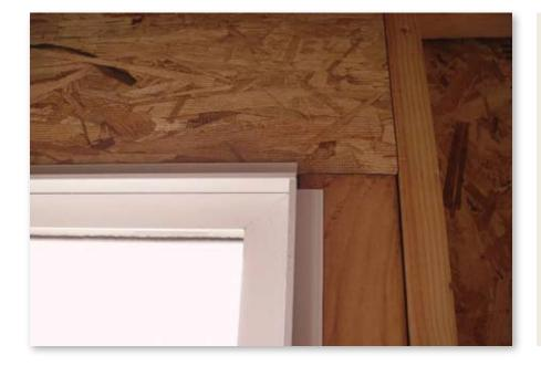
**37.** Place the header and one side jamb extension in place. Line them up so they meet at a flush 90-degree angle, fasten both header and jamb where they meet. Repeat at the other jamb.
