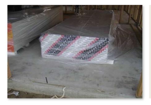
**9.** If drywall is to be stocked in the house, it must be at least 36 inches away from the door opening to provide adequate clearance for the installers to make proper adjustments to the vent panel during installation.
