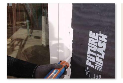
**32.** After the exterior has been fastened in place, Face-caulk the perimeter of the frame where the fin meets the flashing material. All fastener heads and pre-punched holes must be covered with the sealant. Tool the sealant down to insure smooth coverage.
