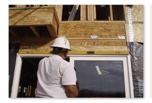
**28.** Using the 4-ft. or 6ft. level, verify that the Door Sill is straight and level. Alternatively, you can do this by checking the Head of the door.
