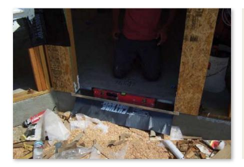
**21.** Place sill pan onto bed of sealant and ensure that it is level.
