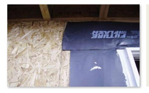
**35.** Apply the flashing at the header so the flashing extends 1 inch past the jamb flashing on each side.
