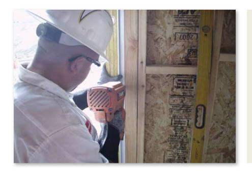
**40.** Use the biggest level that will fit in the opening. Place it against the jamb extenders and fasten the jamb extenders in place, repeat on both sides and the header.
