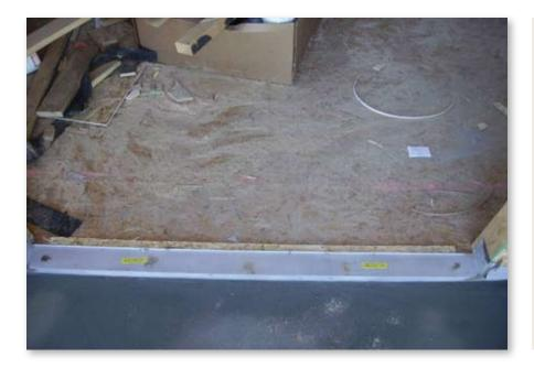
**4.** Sill pans have been installed (where applicable).
