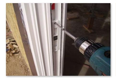
**47.** Once the vent is in the proper position, set the strike plate in place by pre-drilling through the preset holes at the top and bottom of the strike plate and installing the two 3" stainless steel screws (provided with the handle) into the framing.
