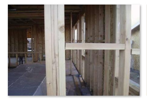
**7.** On open wall framing FIREBLOCKS must be installed and nailed in place.
