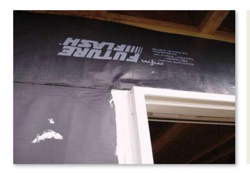
**36.** It is critical that the Head flashing is installed in the weatherboard fashion and embedded in the sealant.
