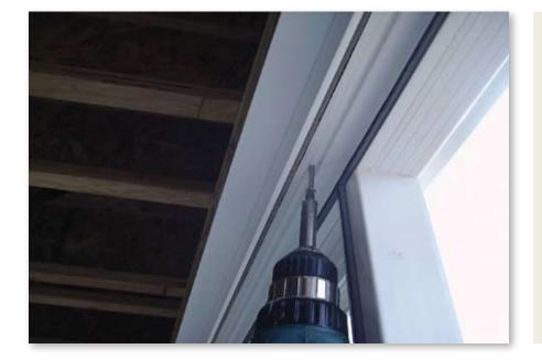
**41.** When the jamb extenders are plumbed you may place 2" screws through the perimeter frame to tighten up any gap that might be present between the frame and the jamb extenders.
