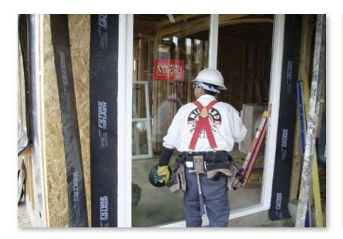
**27.** Lift the door and place into the opening ensuring that you have a good squeeze out with the sealant.
