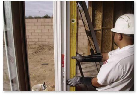
Be sure to place shims between rough frame and the back of the door jamb where the strike plate is to be screwed into.
