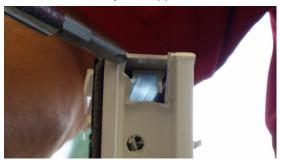
8. Using the self-tapping screw, fasten the new Positive Action Lock to the vinyl sash.
