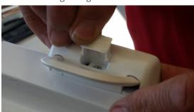
$10. \ \ Reinstall \ the \ sash \ into \ the \ window \ frame \ by \ inserting \ the \ top \ first.$
