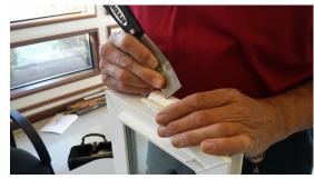
4. Using a Phillips screwdriver, remove the lock screw in the screw port cavity.
