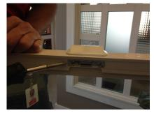
4. Using a Phillips head screwdriver, remove both screws while holding the lock handle in place.
