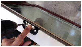
9. Place the thumb lock on operator with the handle turned to the right.
