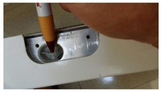
7. Install the new sash lock by inserting it into the sash, making sure the nylon tension strap fits into the slot on the lock operator gear.
