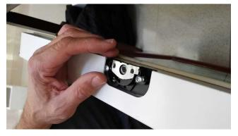
5. Locate the lock gear on the new sash lock.
