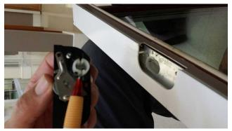
$6. \quad$  Locate the nylon tension strap on the top of the window sash in the aluminum casing
