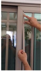
Begin tapping the bead back into the bead groove at the corner. Since it doesn't require a
