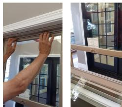
$7. \quad \text{To re-engage the sashes with the jamb, rotate the upper sash until the tilt latches click back into the jamb track.}$
