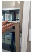
10. Close the bottom sash by pushing down and inward until the lock engages. When the window is closed, it's locked. **NOTE**: Do not pull inward while closing, this might cause the locks to not engage properly.
