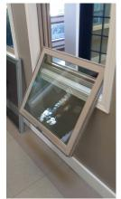
6. Tilt top sash inward. You may rest the top sash on top of the open lower sash.
