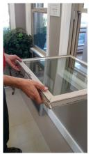
5. Using the pull rail on the upper sash, pull downward until the bottom of the top sash is approximately 6" above the open bottom sash.
