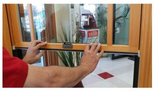
7. Press both tilt latches and tilt the sash to the interior.
