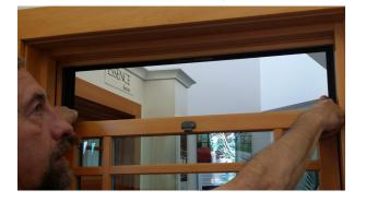
8. To close, rotate the top sash up until it is fully seated in the jamb. Push the top sash up until it is fully closed in to the head of the window.
