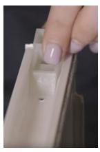
6. Slide the sash to one side to remove.
