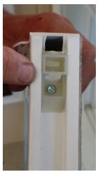
Align the new screw hole with the pre-drilled hole. Fasten the shoe with the screw.
