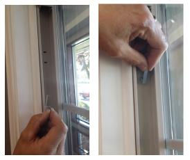
4. Compress the top portion into the top hole until it snaps in the frame.
