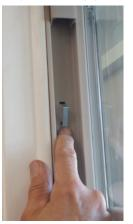
5. Make sure the clip is pushed in flush to the jamb before operating the vent sash.
