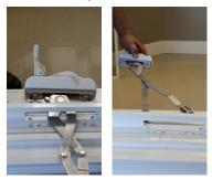
10. Finish by connecting the two operator arm clips to the track guides at the base of the vent sash.
