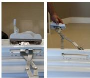
8. Install the new operator into the window frame.
