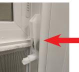
3. Using both hands, lower the carrier so that the locking tab is aligned with the take-out feature. Keep the carrier against the frame at all times while the springs are extended.
