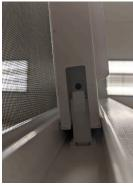
4. Locate the sash cam on right side of the sash near the top. Observe the tab at the top of the sash cam.
