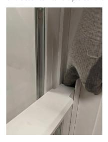
6. While the sash cam is depressed, lift on the bottom left side of the sash. If done correctly, the panel should be pressed into the hand depressing the sash cam.
