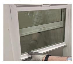
7. Remove hand depressing the sash cam and allow the panel to rotate further, ensuring the cam is not released. Until the panel is removed, the sash needs to be pressed onto the right side of the frame.
