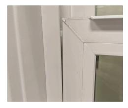
8. Lift the sash so that the bottom rail is higher than the carriers.
