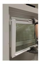
10. Pull the panel to the left, thus releasing it completely from the frame.
