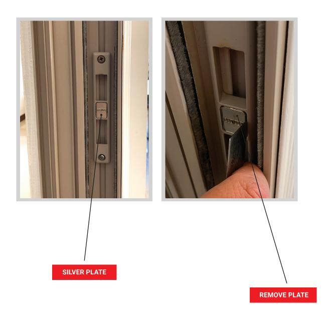
3. Use a Philips head screwdriver to remove the screws on the top and bottom of the strike. (This will allow you to loosen center screw under silver plate that will allow you to move strike up or down.)
