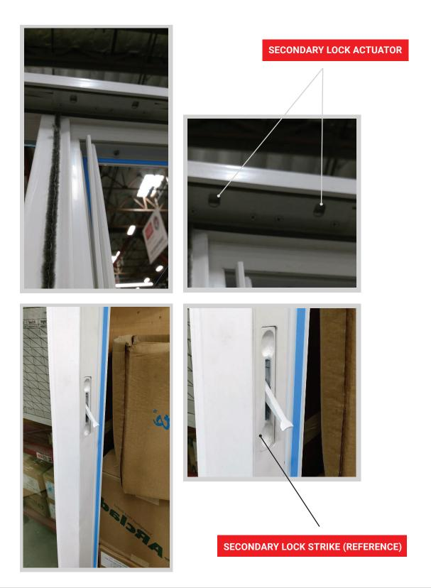
6. Open panels and loosen 2 factory installed screws holding shoot bolt strikes at both head and sill. There will be four of them total. The strikes are slotted so they can be moved into position.
