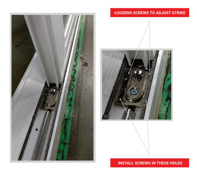
7. Close passive panel. Engage shoot bolt into strike at sill, center shoot bolt in strike. Open panel and install 2 screws in the rear strike holes that previously did not have screws in them. Tighten both screws and then tighten the 2 original screws in the strike. Retract shoot bolt and open and close panel to make sure engagement is smooth.
