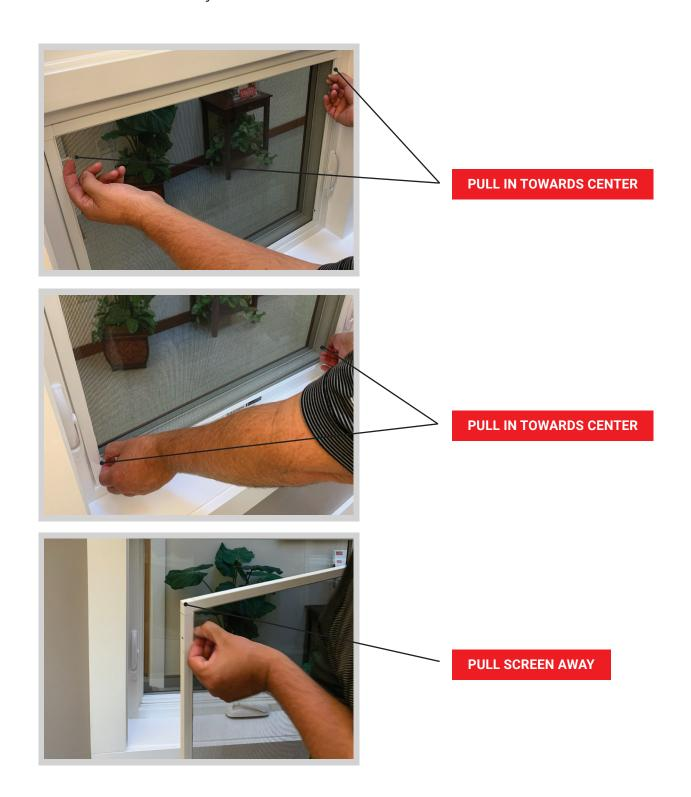
6. To reinsert, pull the pins in, insert the bottom. Pull the top pins in and insert the top.
