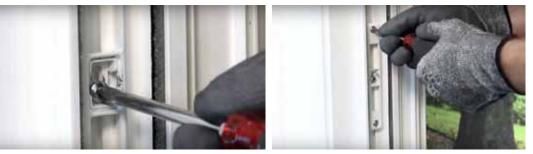
6. The strike plate can be moved up and down accordingly. Once in proper alignment, reinsert the screws and the strike plate.
