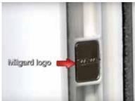
4. Using a putty knife, remove the strike plate to expose the adjustment screw.
