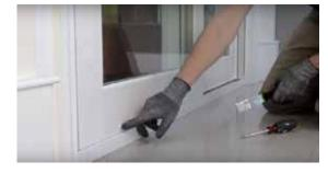
2. Using a stiff putty knife, remove these plug covers. The screw ports allow access to Phillip head screws that raise and adjust the door.
