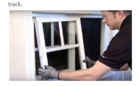
2. On the bottom of your window there are two assemblies containing vinyl wheels. Each assembly has two position for each wheel. Using a flat head screwdriver remove the wheel by snapping it out of the wheel casing.
