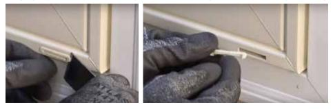
8. Use the pipe cleaner to clean the weep-hole of access debris. Place the weep-hole cover back into the weep-hole.
