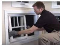
3. Using a putty knife, lift up and remove the track. Clean the track using a non-abrasive cloth, soap and water. It is important to avoid abrasive chemicals.
