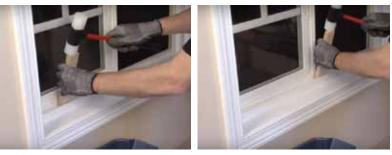
5. Install the sash from the top, slide it in from the bottom.
