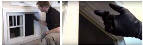
2. Lift up on the sash from the bottom, pull out and down to remove the sash. You may notice that moisture and debris is present in the window track. This is normal.
