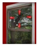
1. Glass is measured with the width measurement first and the height measurement second. Place the tape measure at one end of the glass and extend to the other end of the glass. Look carefully at the tape measure and include the glass measurement accurate to an 1/8th of an inch.
