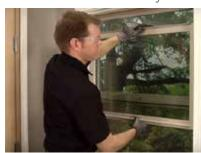
6. Push in both of your takeout clips, bring down the sash and reinstall the sash stops.
