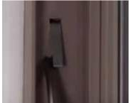
2. Remove the sash stops, which are located in the top corners of the window.
