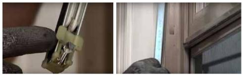
5. Push the top portion up and the tab goes on the outside of the balancer.
