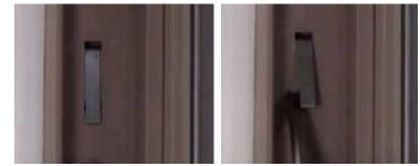
2. Remove the sash stops, which are located in the top corners of the window. Slide the sash up until you feel it disengage. You will want to make sure both side catch on the take-out clips. Once they catch, you will want to be able to see the bottom of the spring-loaded balancers and you know you are past the engagement point. Slide the sash to one side and remove.
