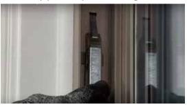
6. Next, reinstall the sash. Place the sash above the bottom of the balancer. Line up the sash, push it in. Make sure you have clearance on the other side and balance it back and forth until you feel both tops catch. Slide the sash down about an inch or two. Make sure you do not see the balancer or any metal on either side of the spring. Then push in both of your take out clips and bring down the sash. Finally reinstall the sash stops.
