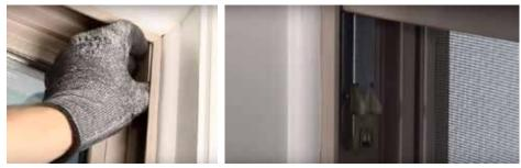
3. To remove the balancer, push it down and slide it back up. (The balancer is spring-loaded so use caution when removing.)
