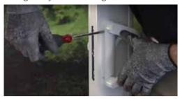
2. Once you have removed the screws, the handle slides out which gives you access to the snib which also slides out.
