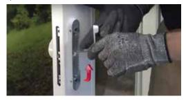
4. With the new snib in place, put the handle back on and secure it with the screws. Check the snib operation to ensure that it is installed correctly. Shut the door to ensure the lock engages.
